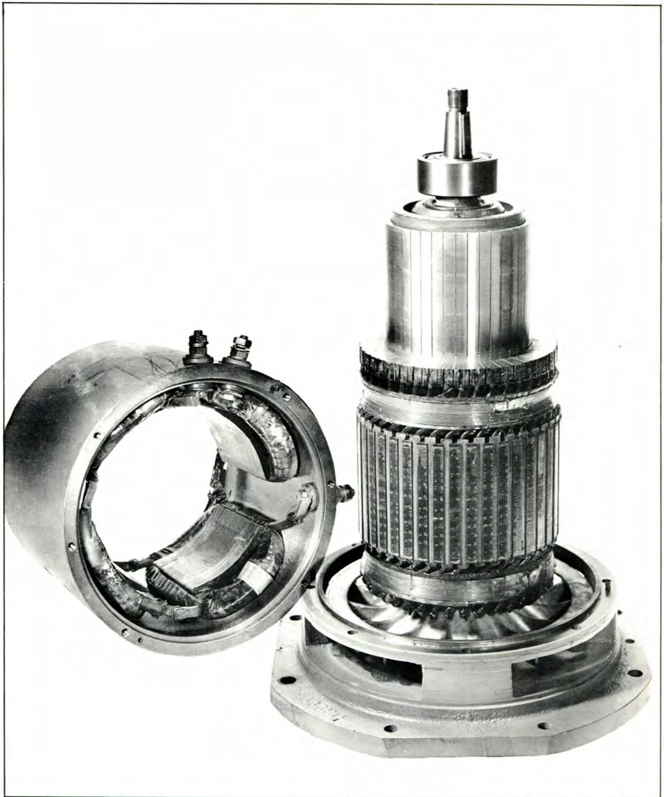
Plate 7562. Typical Drive Motor Assembly
